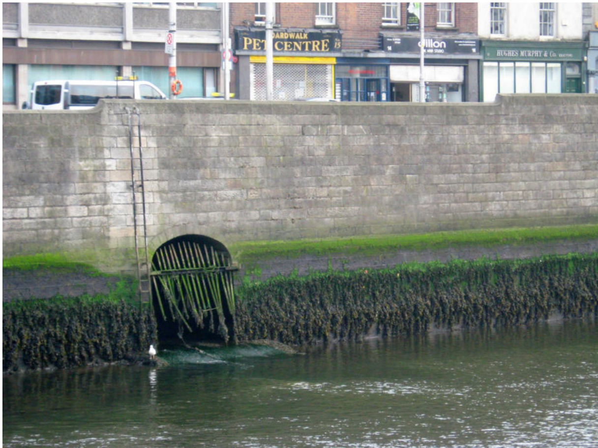
The grate where the Poddle flows into the Liffey, at low tide, at Wellington Quay.
