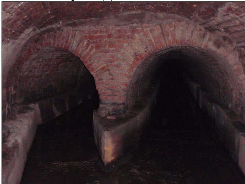
The main culvert under Dublin Castle.
